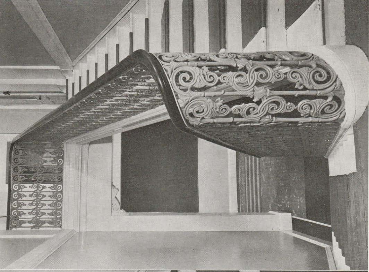
20. 9 St. Leonard's Place, staircase.
