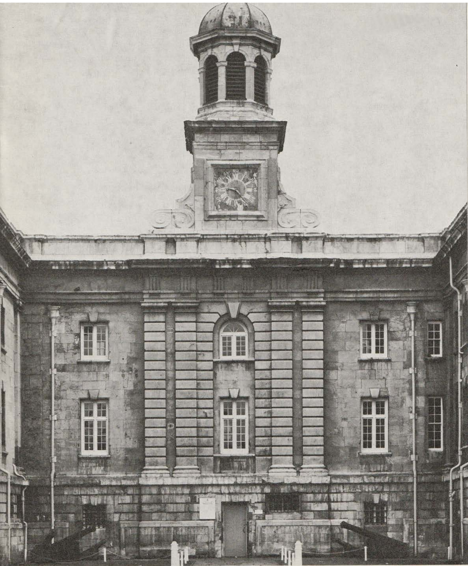
1. Debtors' Prison, Castle Yard. The designer of this handsome building is not known. It was erected in 1701-5 and is characteristic of the English baroque style; our picture shows the central block.
